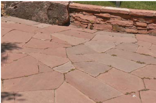
Typical sand-set flagstone patio with retaining wall
