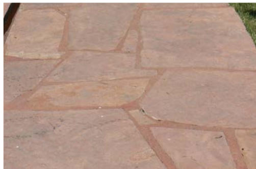
Colored mortar with loose jointing
