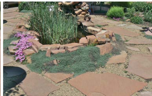
Pallet-sized flagstone widely spaced in pea gravel
