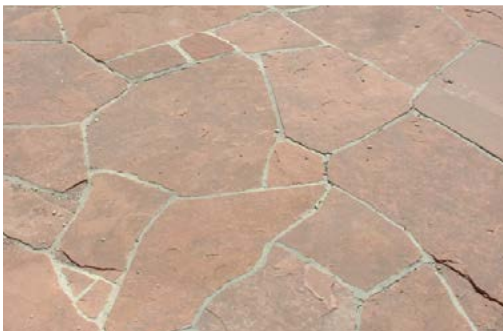
White mortar with tight jointing
